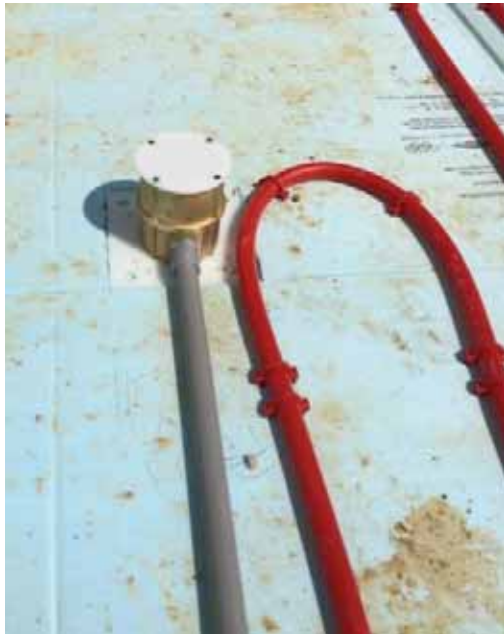
Sensor socket before concrete
