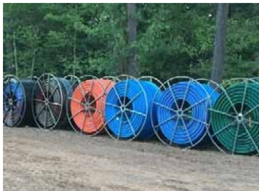
PCD: HDPE Conduit for fiber optic
