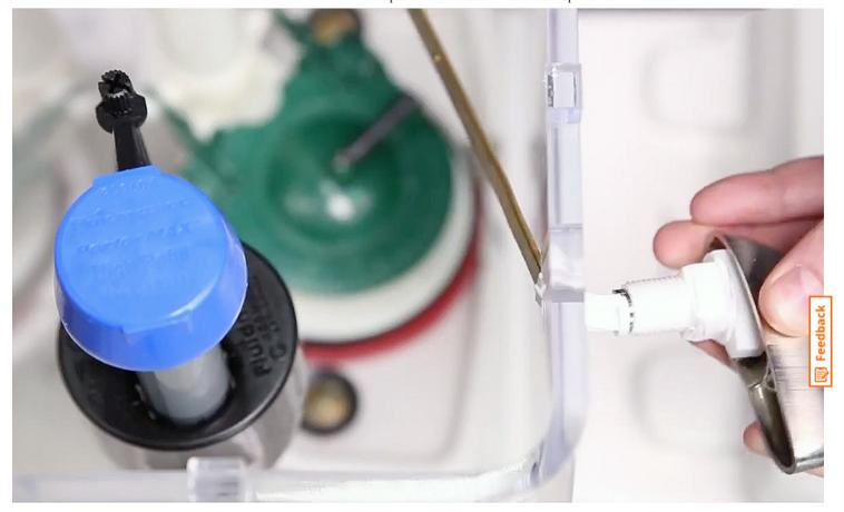
With the mounting nut removed, slip the lift arm through the hole in the tank to remove the old handle.
