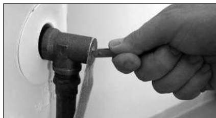
Figure 45 - T&P Relief Valve.
