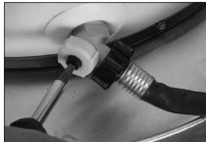
Figure 20 - Draining the old water heater.
