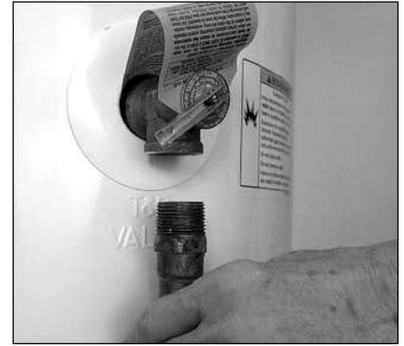
Figure 21 - Removing the T&P Relief Valve discharge pipe.
