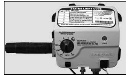
Figure 56 - Gas control/valve with threaded pipe.
