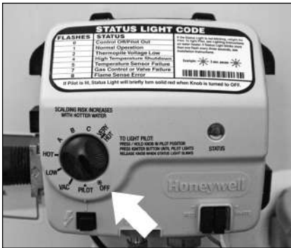
Figure 40 - Turn gas control/temperature knob OFF.
