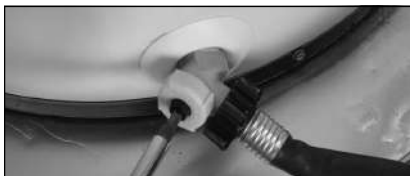
Figure 42 - Draining the water heater.
