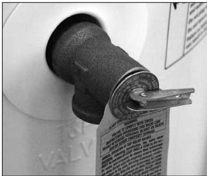
Figure 25 - Temperature and Pressure Relief Valve
