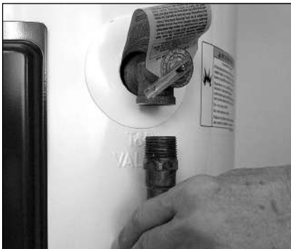
Figure 11 - Removing the T&P Relief Valve discharge pipe.
