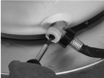
Figure 10 - Draining the old water heater.
