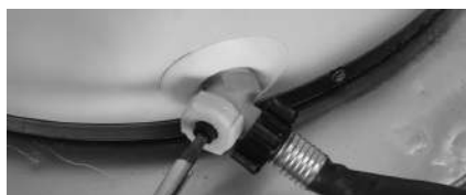
Figure 26 - Drain Valve
