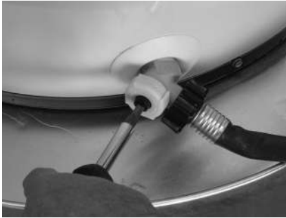
Figure 10 - Draining the old water heater.
