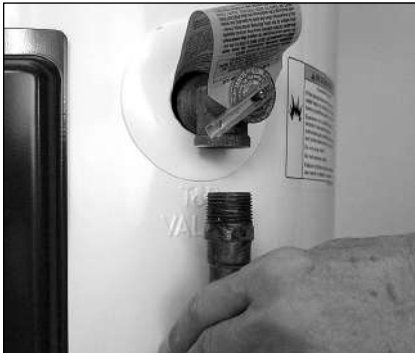
Figure 11 - Removing the T&P Relief Valve discharge pipe.
