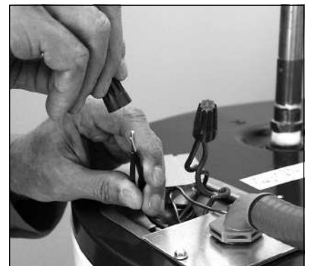
Figure 19 - Connecting the electrical wires.
