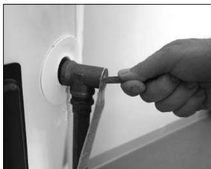
Figure 38 - T&P Relief Valve
