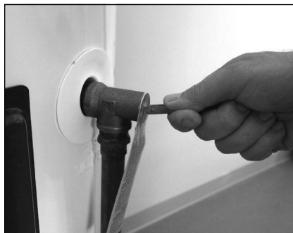
Figure 38 - T&P Relief Valve
