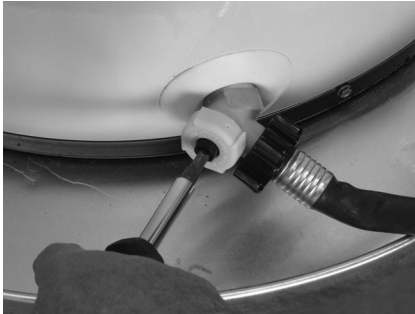
Figure 10 - Draining the old water heater.
