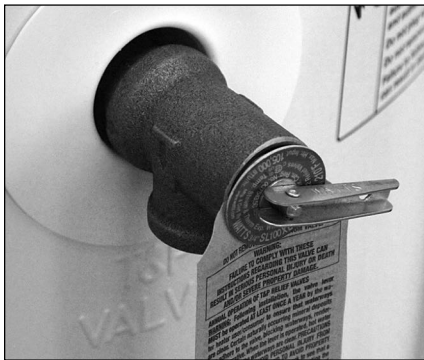
Figure 25 - Temperature and Pressure Relief Valve
