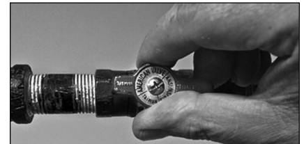
Figure 58 - Gas valve in "on" position.
