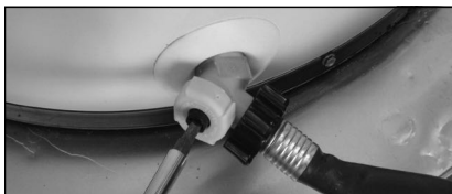
Figure 42 - Draining the water heater.
