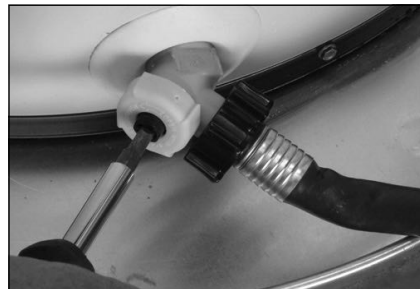
Figure 20 - Draining the old water heater.
