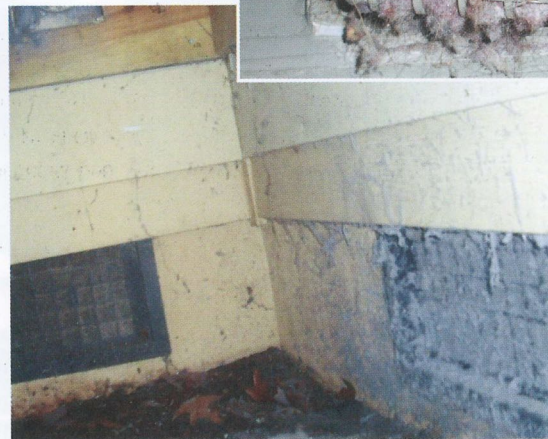
Photo 7. Wonder what the inside of the duct looks like?
