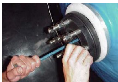
Step 5: Screw flange adaptor on assembly. Be sure O-ring is attached and sealed properly to adaptor.
