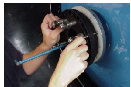
Step 6: Use backing flange to connect distribution system to 6" flange. Now remove extension.
