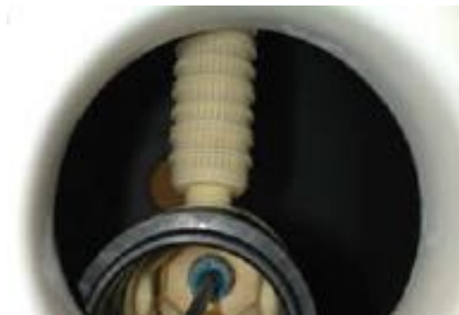
Step 4: Screw all laterals in hub while still holding extension.
