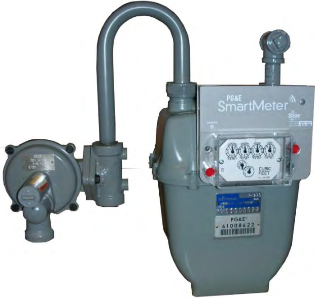
Figure 2-14 Typical Residential Gas Meter Connection
