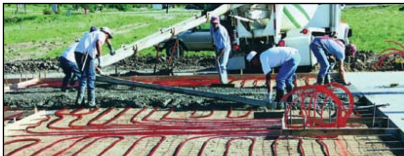
Figure 11.1 – Radiant Floor Heating Piping
