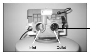
Insert Flow Straightener into outlet side of valve. The pointed side of the flow straightener is to face outward.
