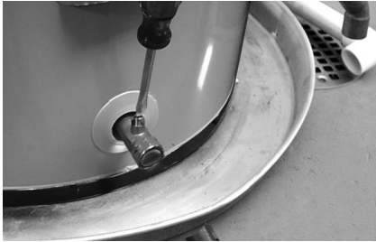
Figure 10 - Draining the old water heater.
