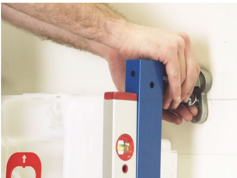
7 - Place the fixing brackets at the top of the frame.
