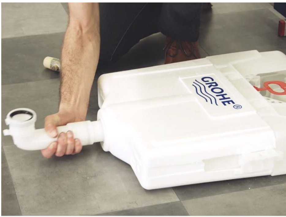
3 - Place the vertical flush pipe on to the underside of the cistern
