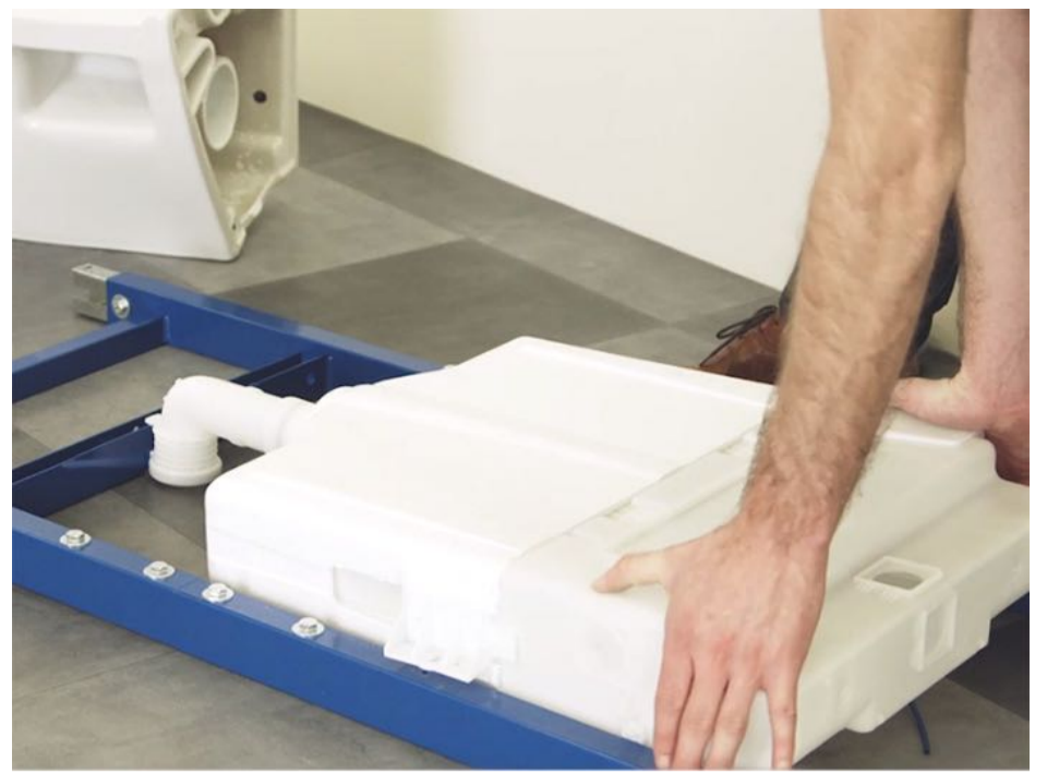
4 - Secure the cistern in to the frame. First place the elbow of the flush pipe on the frame, and then press down on the cistern to clip it into place.
