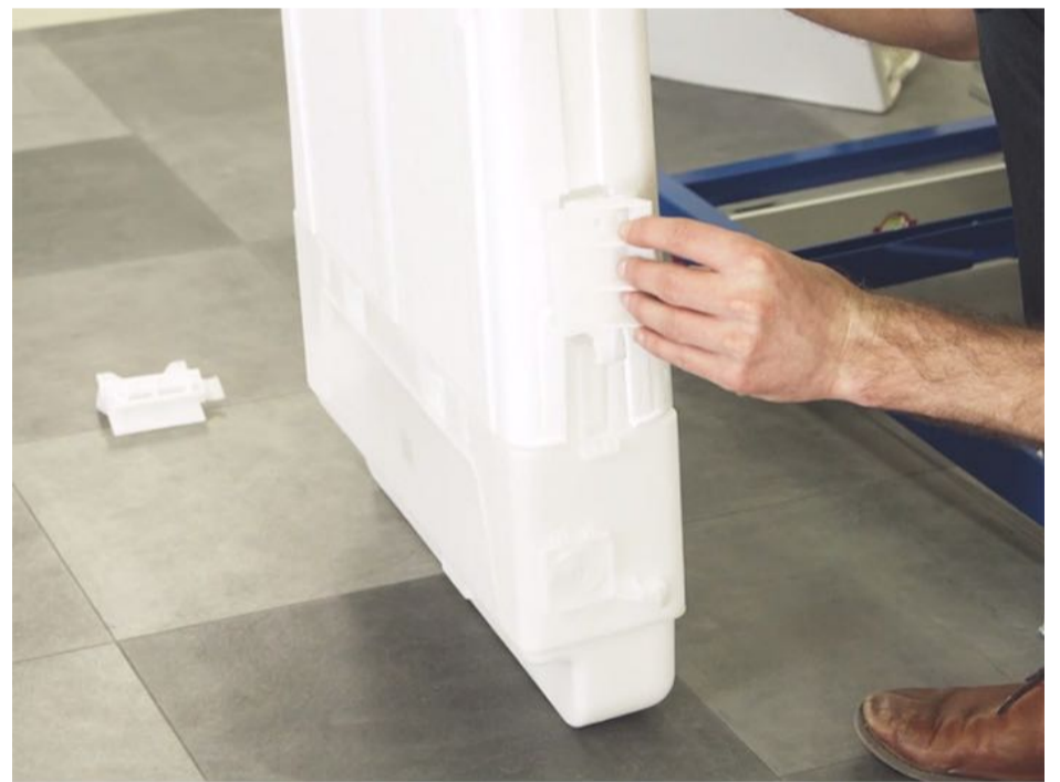
2 - Slide the 2 fixing mounts onto the sides of the cistern making sure they are fitted securely.
