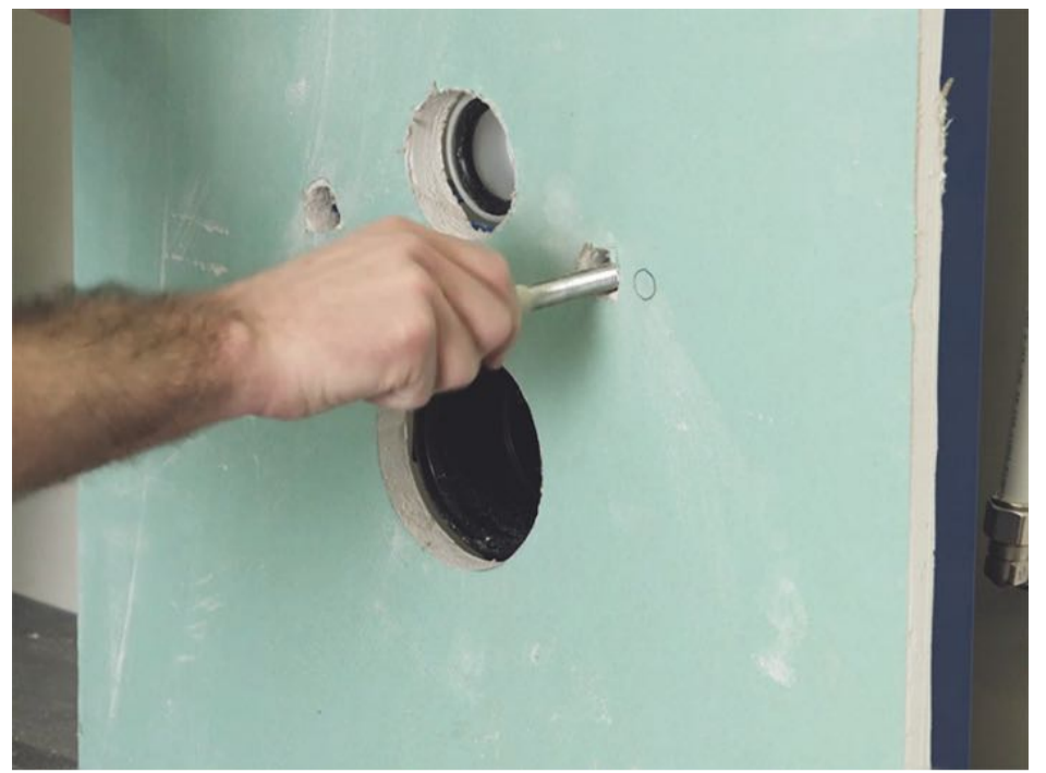
2 - Screw in the threaded rods with the cardboard covering in to the frame
