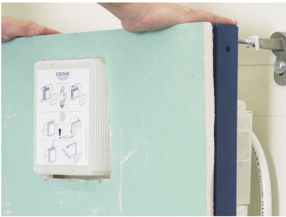
1 - Cut the covering panels to match the unit's openings and sides.
