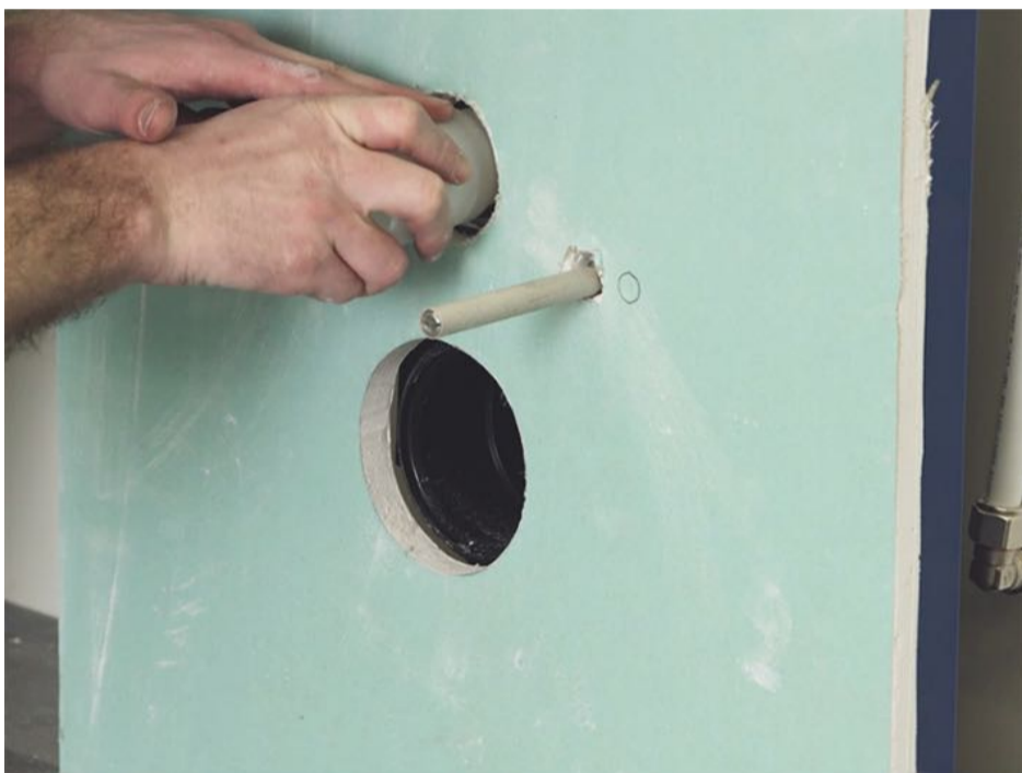
3 - Place the cut-out templates for the waste and flush pipe.
