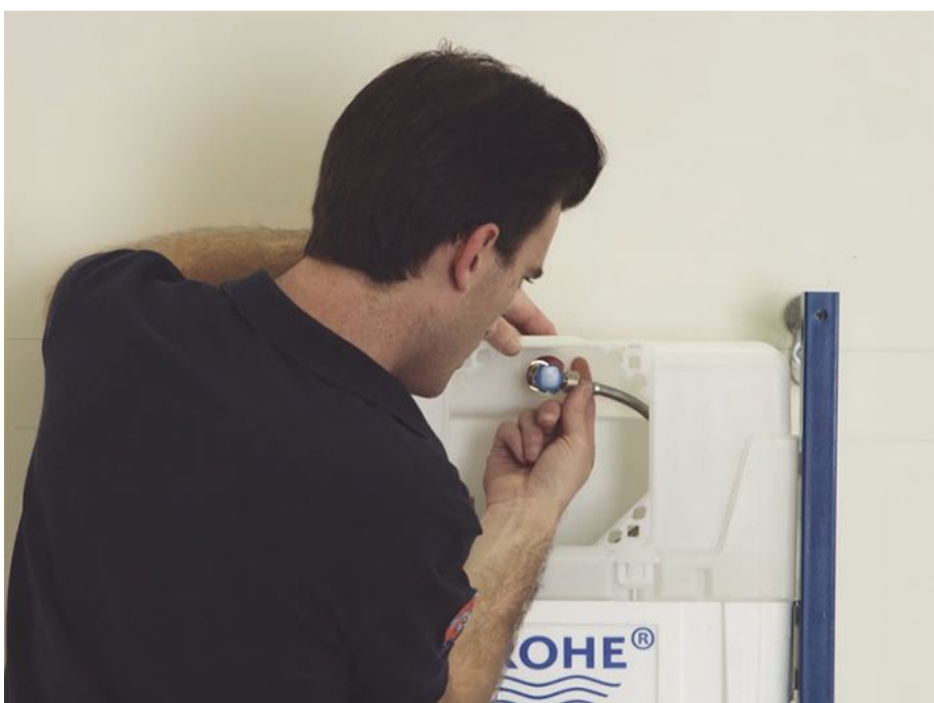
5 - Connect the internal flexible water inlet hose to the stop valve.
