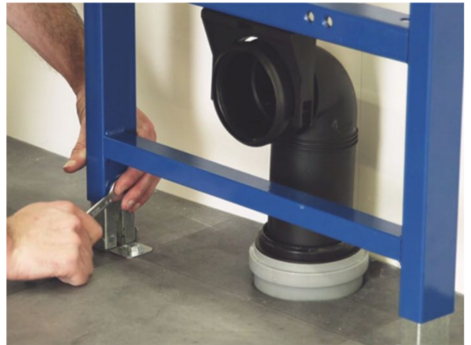
6 - Adjust the level by loosening the adjustment bolt on one of the feet using a 13 mm wrench, then tighten the screw. Make sure the screw is firmly tightened on the other foot.
