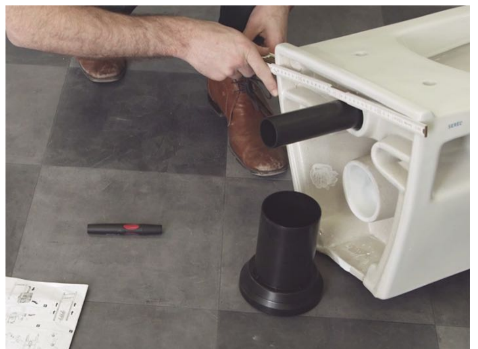
2 - Place the pipes on the bowl and mark the pipes where they
