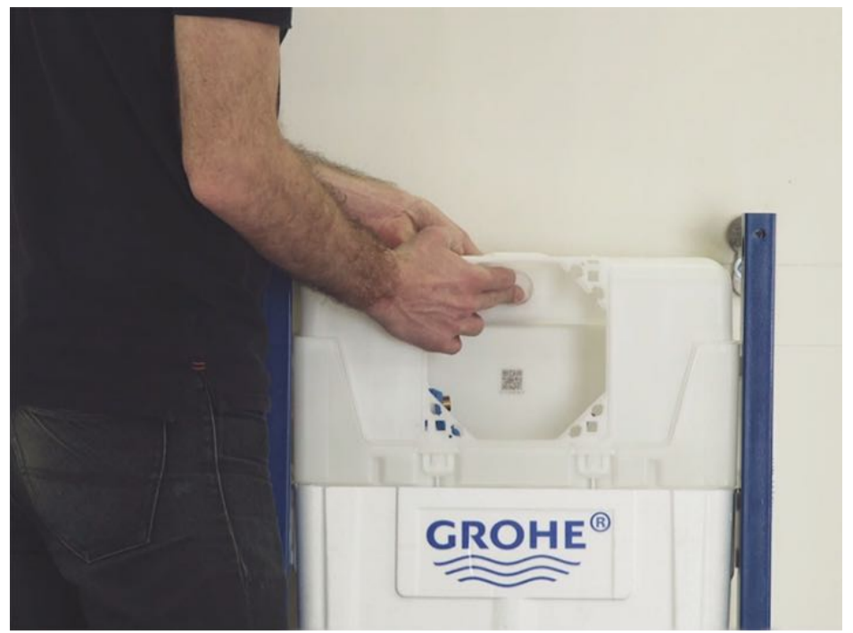
2 - Remove the cover to access your cold water connection
