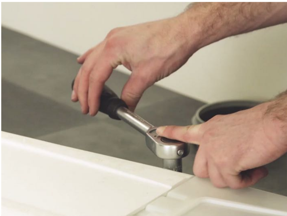
5 - Use a 10 mm ratchet wrench to attach the fixing mounts on the frame.
