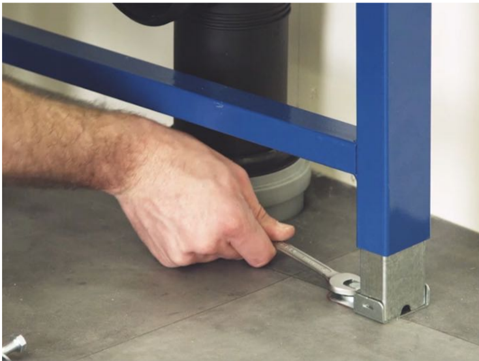
5 - Secure the feet using a 13 mm wrench. Make sure the frame is level horizontally.
