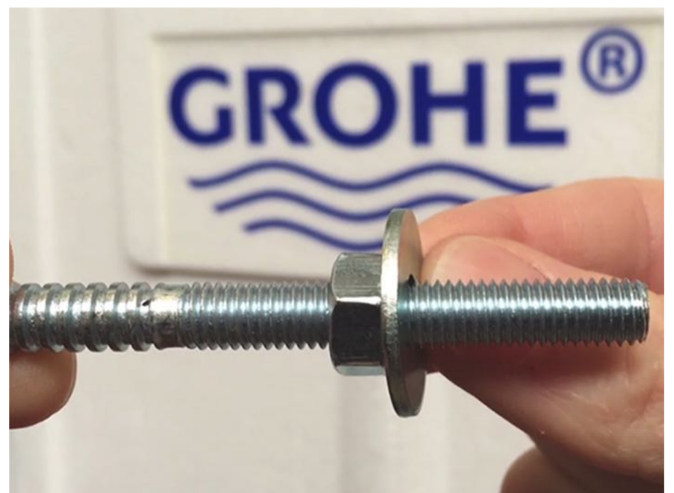
8 - On the threaded rod, place 1 nut, 2 washers and 1 nut.
