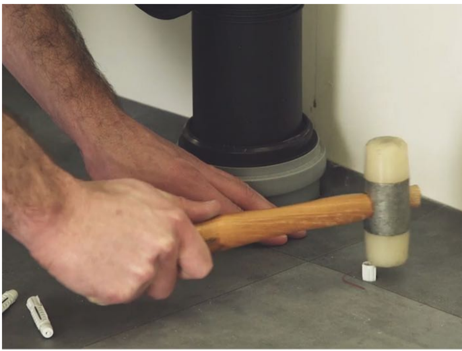
3 - Drill holes into the floor using a 12 mm drill bit. Insert the rawl plugs
