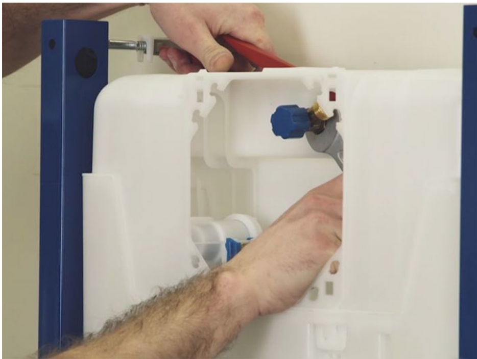
3 - Attach the exterior part of the stop valve to your cold water connection using a 22 mm open-end wrench and a pipe wrench. This assembly must be made without using a seal.
