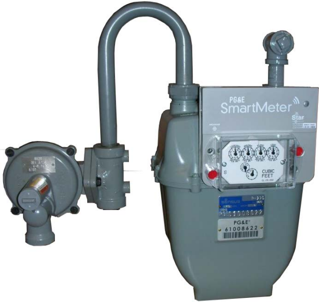
Figure 2-14 Typical Residential Gas Meter Connection
