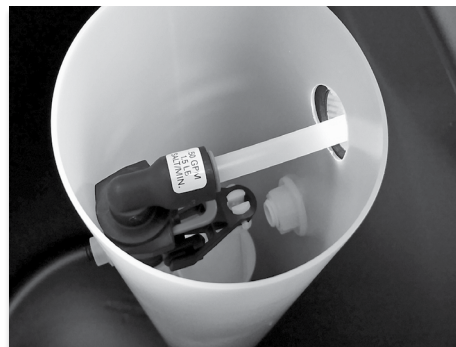
Connection at Brine Safety Float in brine tank
