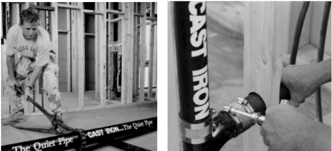
Figure 4—Assembling Hubless Cast Iron Soil Pipe Is Literally a Snap. Only Two Tools Are Required, a Pipe Cutter and Torque Wrench.
