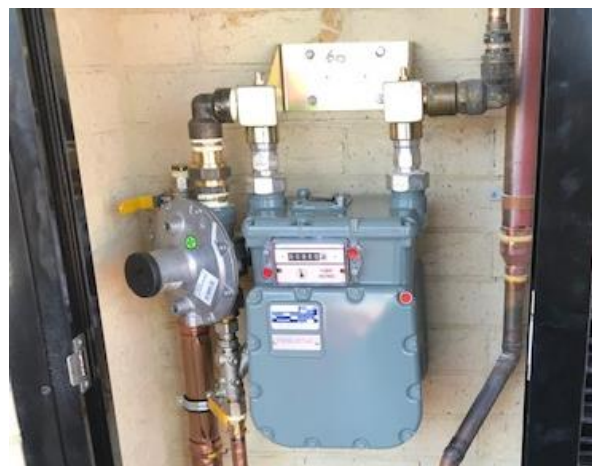
Right: AL12/AL18 Meter Bracket
