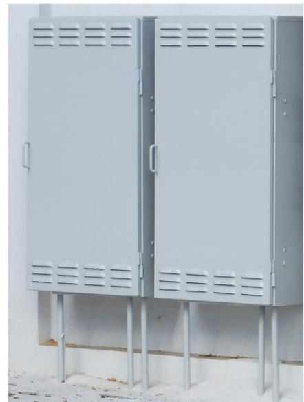
2 x Double Boxes Installed
