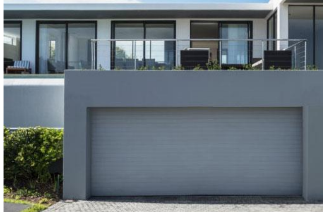
Not Acceptable – Concealed under Carport
