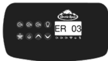
ER03 - Spa Over Temp
