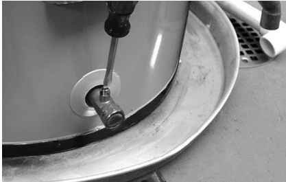
Figure 10 - Draining the old water heater.
