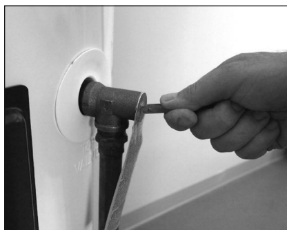
Figure 38 - T&P Relief Valve
