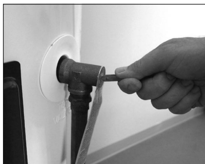
Figure 38 - T&P Relief Valve
