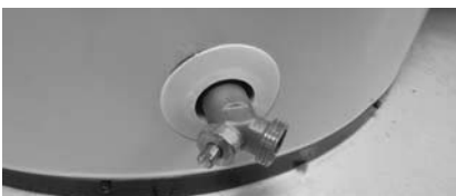
Figure 42 - Drain Valve
