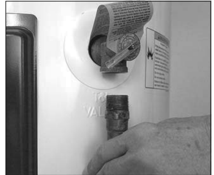
Figure 13 - Removing the T&P Relief Valve discharge pipe.
