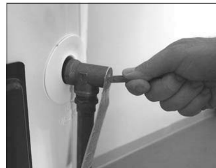
Figure 46 - T&P Relief Valve
