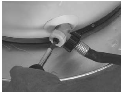
Figure 12 - Draining the old water heater.
