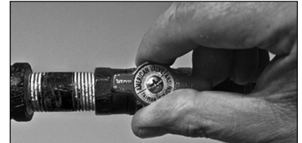
Figure 58 - Gas valve in “on” position.
