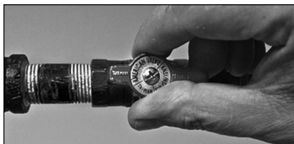
Figure 32 - Gas valve in "on" position
