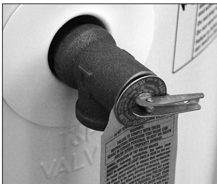
Figure 25 - Temperature and Pressure Relief Valve
