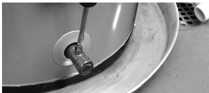
Figure 42 - Draining the water heater.
