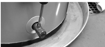
Figure 42 - Draining the water heater.
