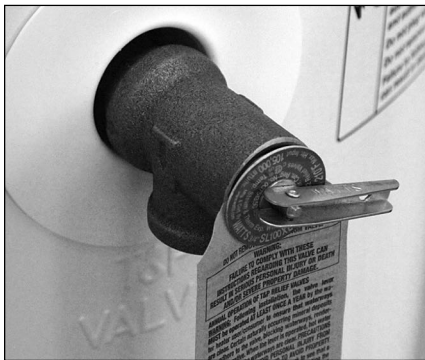
Figure 25 - Temperature and Pressure Relief Valve
