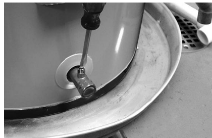
Figure 20 - Draining the old water heater.
