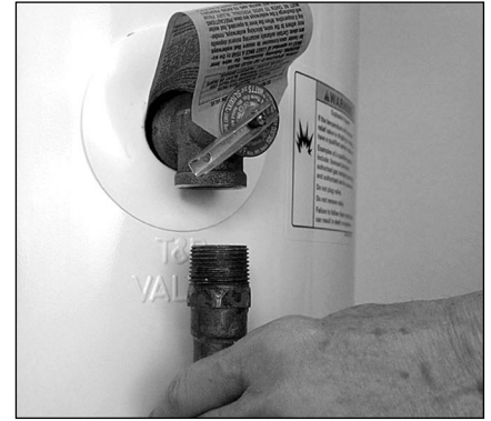
Figure 21 - Removing the T&P Relief Valve discharge pipe.
