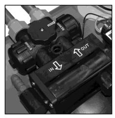
Figure 9: Bypass Valve
