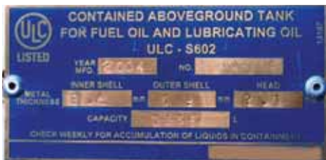
ULC certification plate, standard, double-wall, steel above-ground home-heating oil tank.
