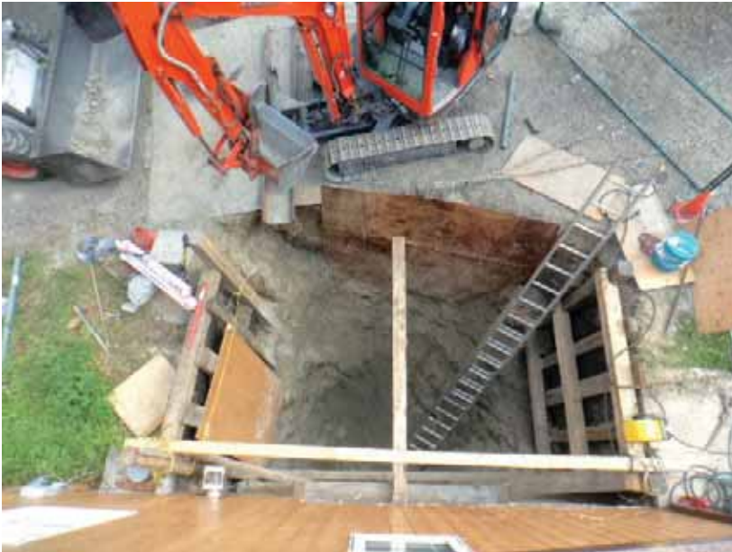
An overhead view of a residential fuel oil spill being remediated.
