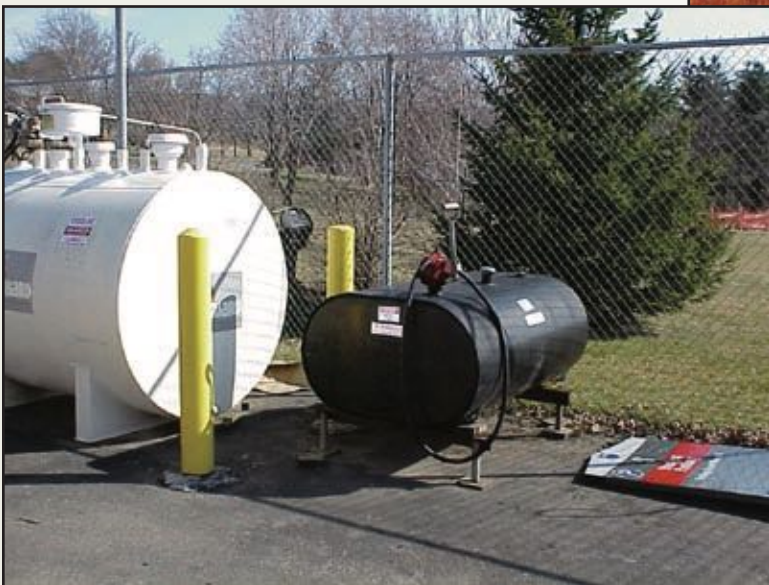
Above: The black indoor tank is being used outdoors.
