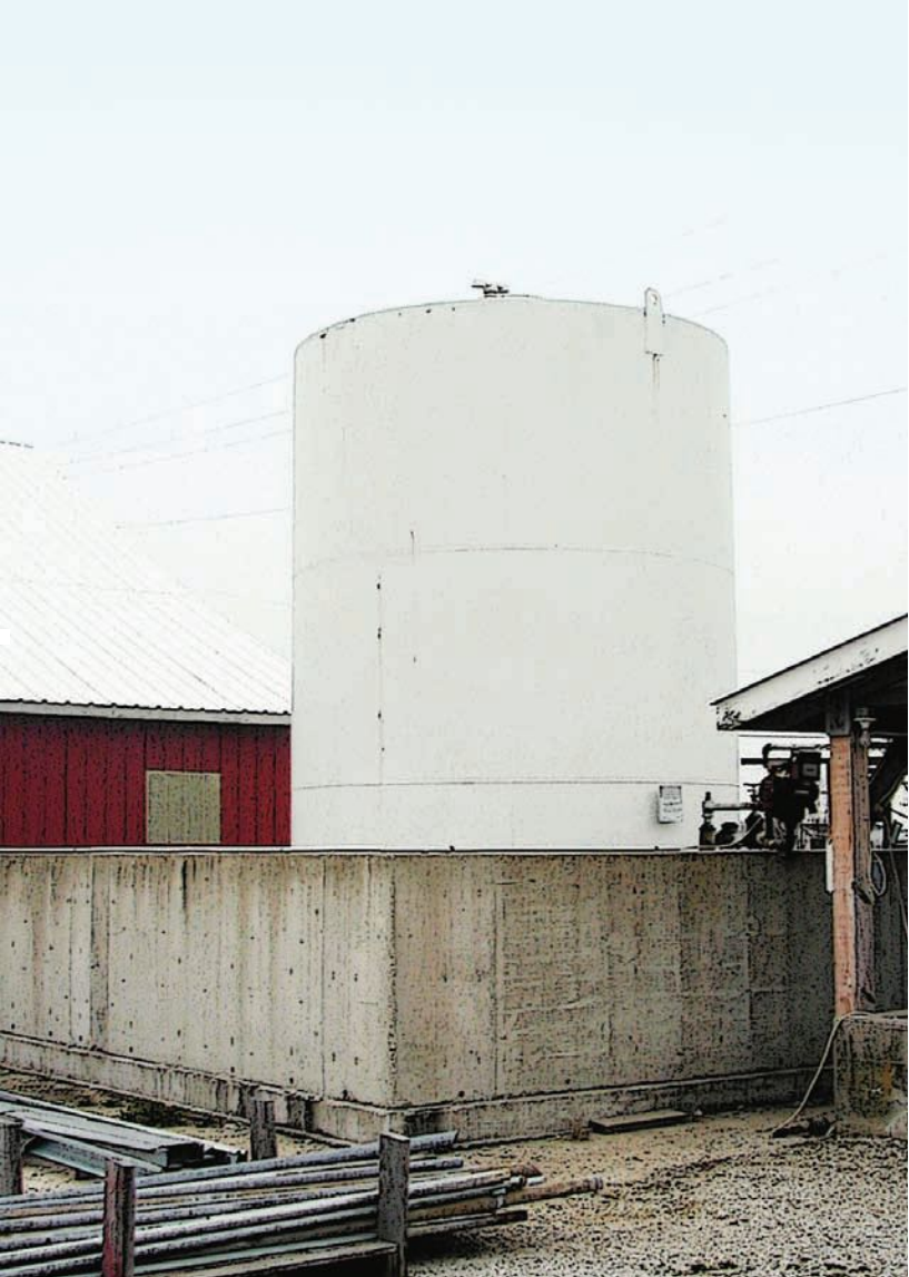
Above: Large diesel tank in containment.
