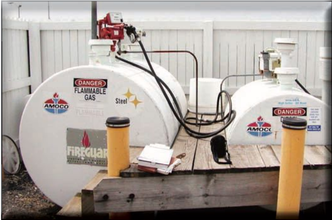
Top left: A platform provides access for filling tanks.
