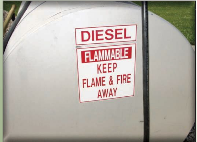
This tank is marked with large lettering indicating the product type and warning the user about hazards associated with the product.
