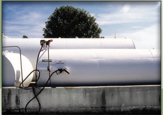
Top left: Notice the curbed containment beneath this heating oil tank.
