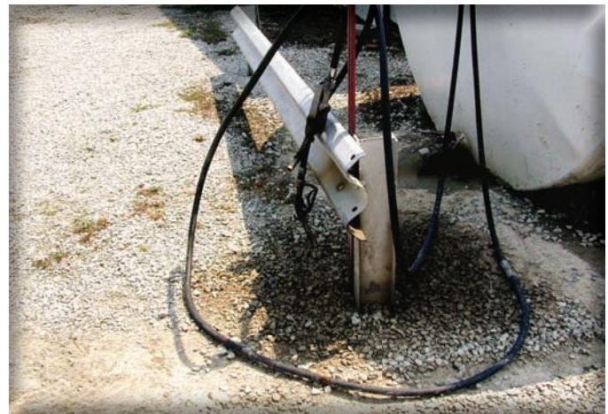
Automatic nozzles do not always shut off. Require anyone fueling equipment to remain at the fuel nozzle.
