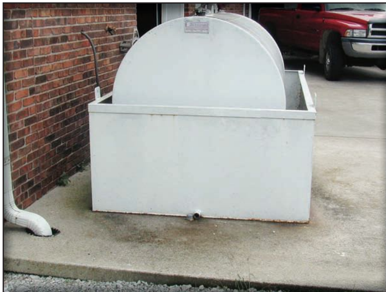
This tank has been painted to discourage erosion. However, notice that its content is not identified. Also notice that the plug to the secondary containment has been removed!
