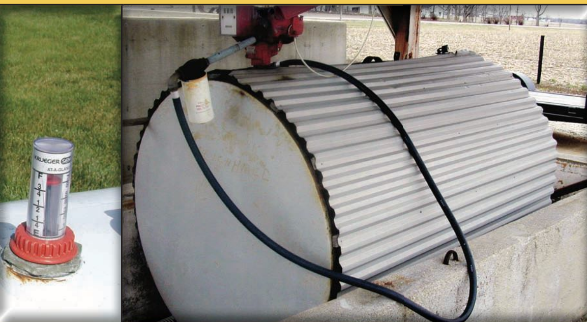
This tank under roof is wrapped to deflect heat, helping to reduce vapors.
