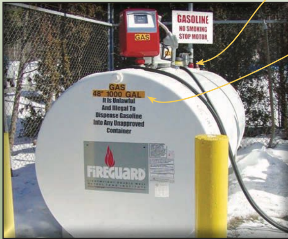
Left: The tank is equipped with a fuel level indicator. Note that 48 inches of fuel is 1000 gallons.
