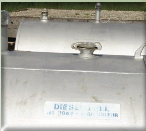
The labels on these tanks are faded and worn—some even partially torn off—making content identification difficult.
