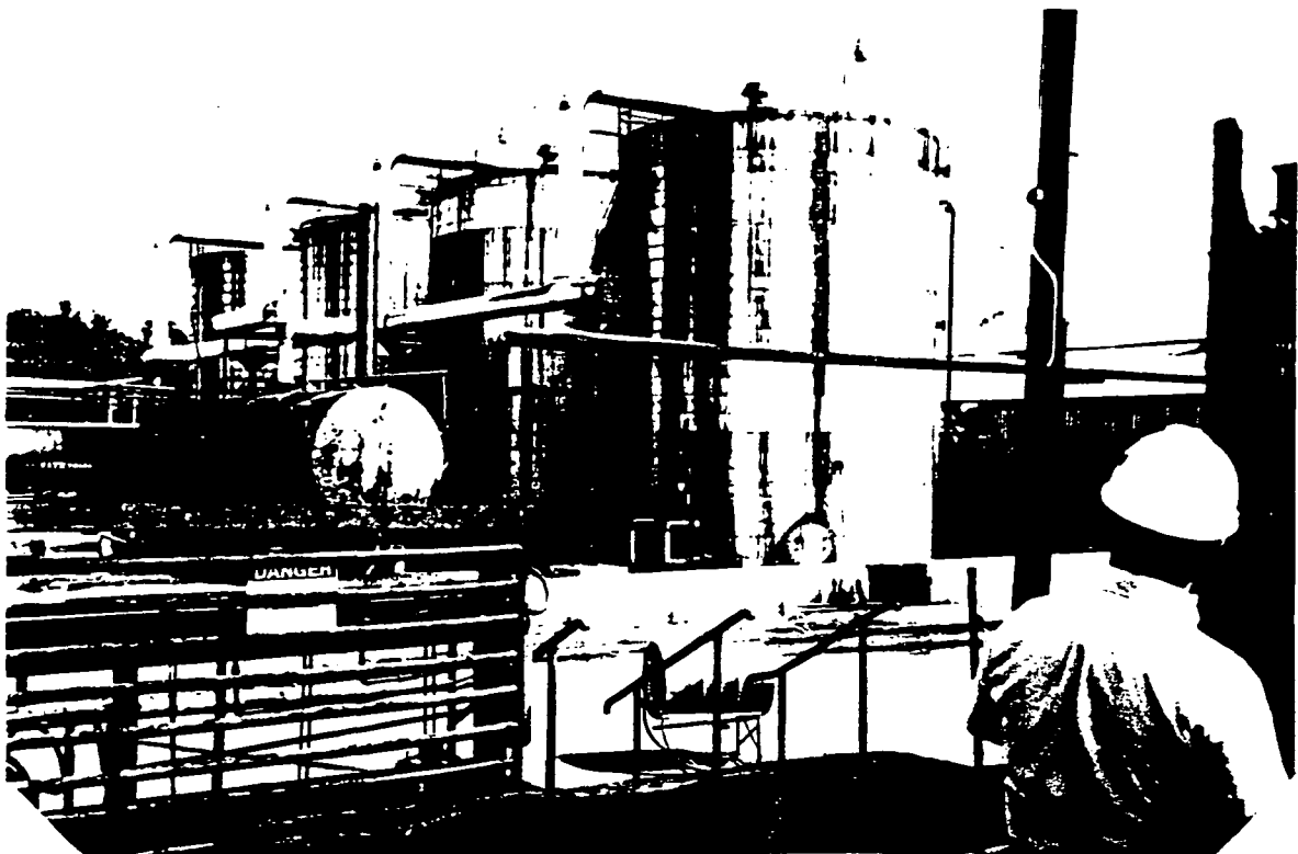
View of four creosote working tanks and scrubber used to control blow back vapors.
