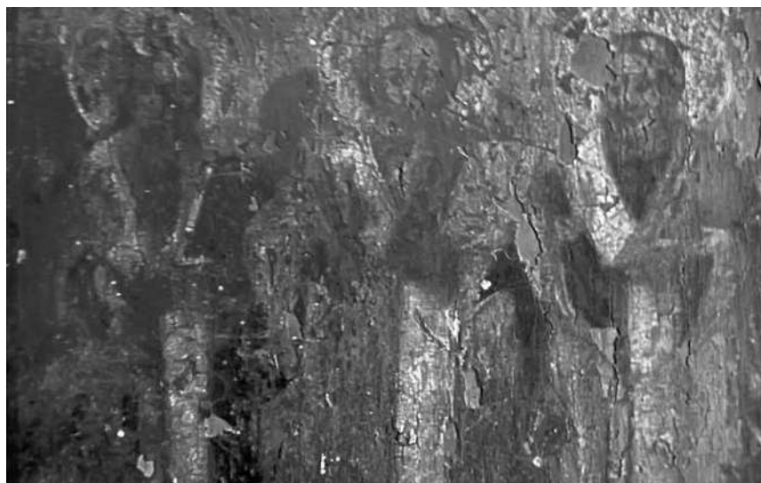
Figure 3. Cracks, separation, multiple and profound gap sin the paint layer to support wood nun even small.
