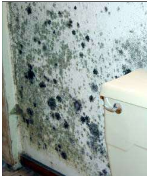
Many mold colonies growing on dry wall in a residence. (Image courtesy of Dr. Chin S. Yang of P&K Microbiology Services)
