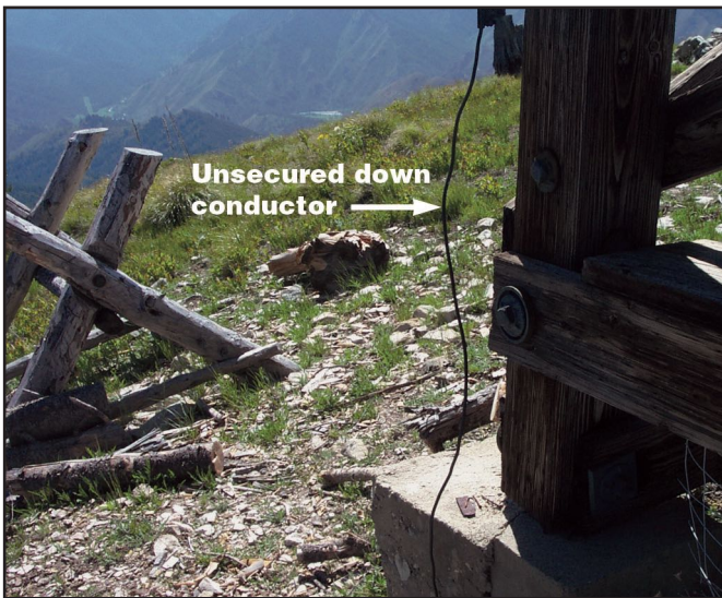
Figure 2—Down conductors should be secured to the structure and not permitted to move or flex.
