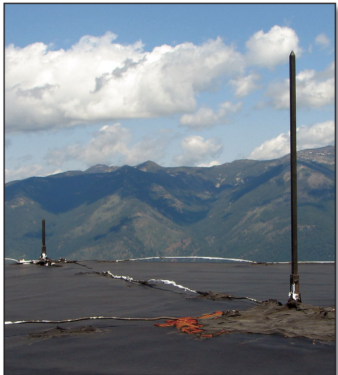
Figure 1b—These proper air terminals are constructed of ½-inch diameter copper rods and have at least two conduction paths to an earth ground.
