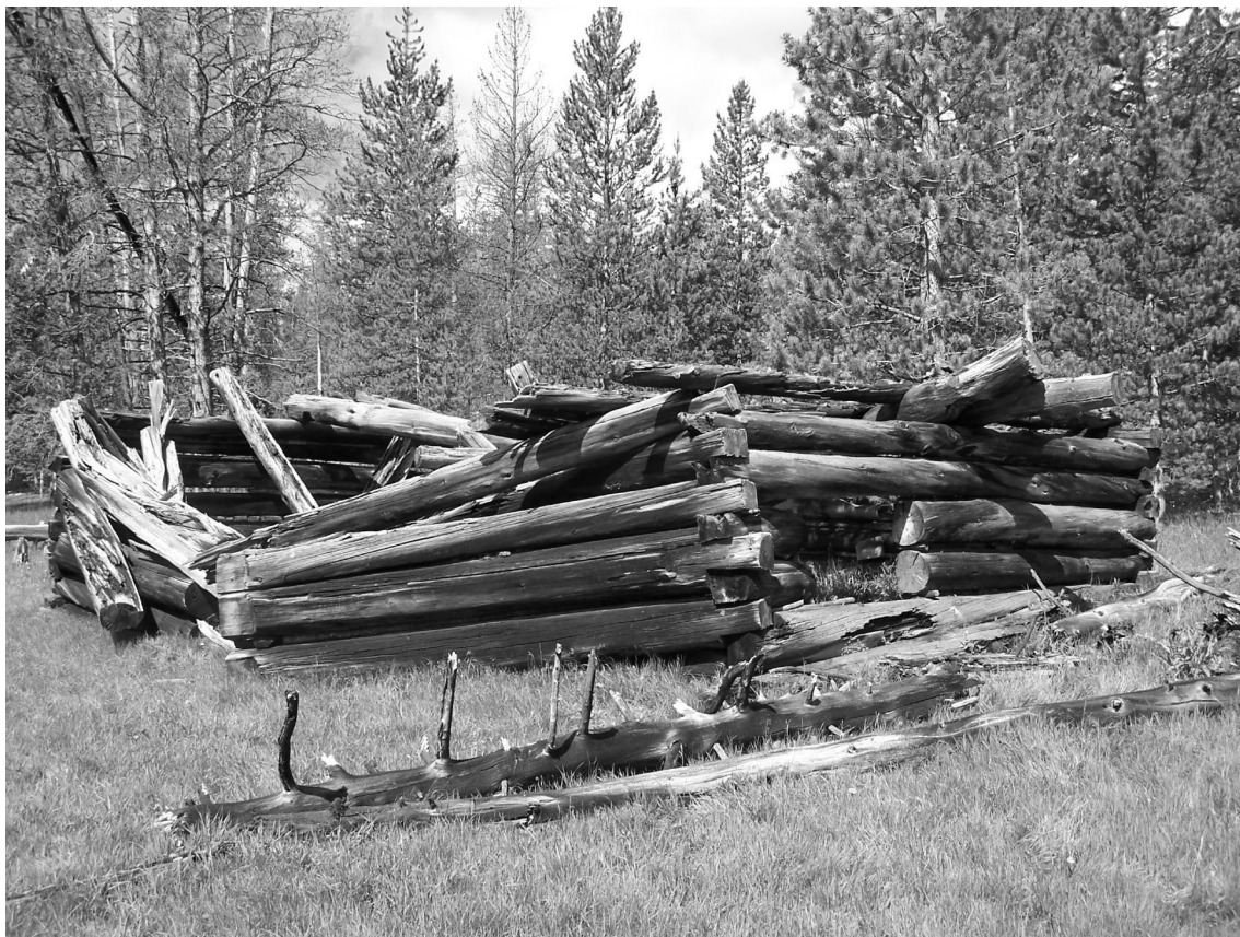
Figure 2. Collapsed log cabin barn that once held the four to six horses common to a tie camp during the 1910s–1920s, near Black’s Fork River.
