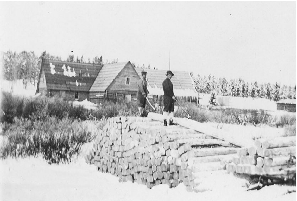
Figure 5. Mill Creek Commissary in background, with tie cutters piling, or banking, finished railroad crossties to be floated downstream in the spring, ca. 1912–1913. The splash dam would be a few hundred yards to the right (north).
