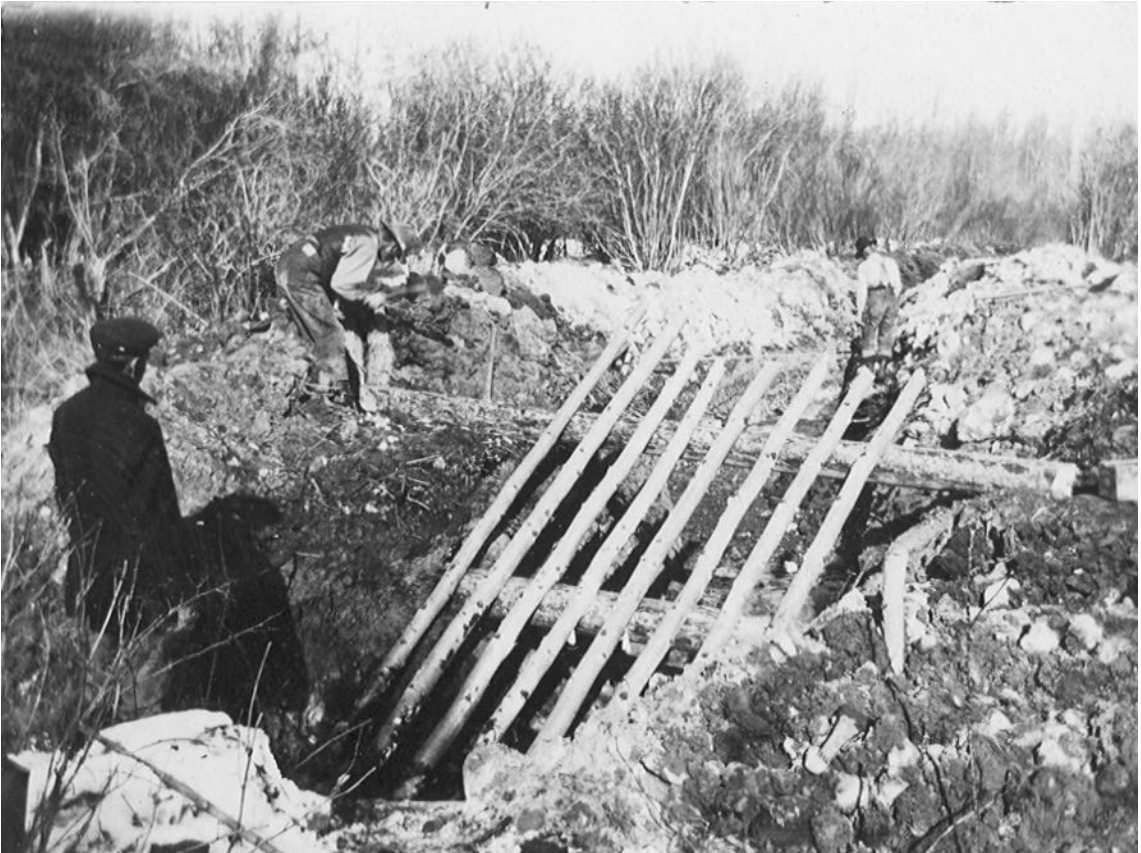
Figure 3. Standard Timber Company crews constructing aspen and willow cribbing to protect irrigation canals from being filled with railroad crossties in the Mill Creek area, ca. 1912–1913.
