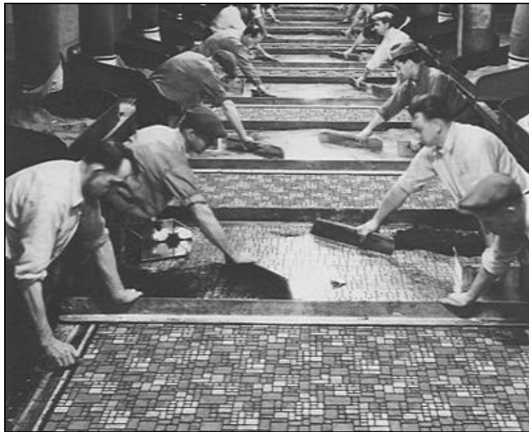
Figure 18. Workers with Embossed Inlaid Linoleum (after Mehler 1987:153)
