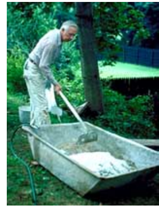
The dry materials must be mixed thoroughly before adding water to make the stucco. Photo: NPS files.
