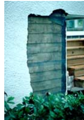
The stucco will be applied to the wire lath laid over the area to be patched. Photo: NPS files.
