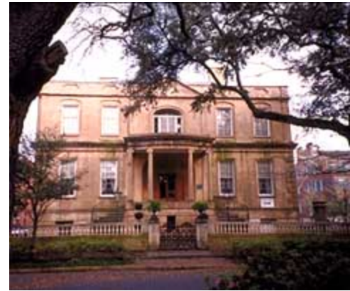
The stucco on the early-19th century Richardson-Owens-Thomas House in Savannah, Georgia, is a type of natural cement. Photo: NPS files.
