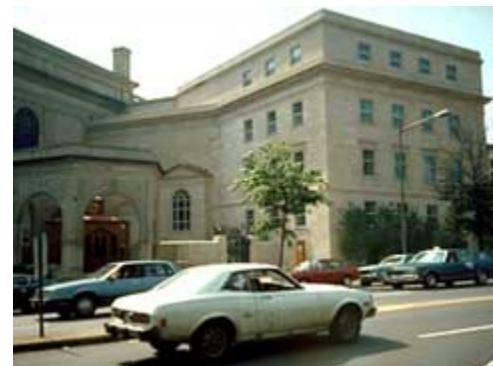
The new addition on the right is stucco scored to imitate the limestone of the historic building on the left. Photo: NPS files.
