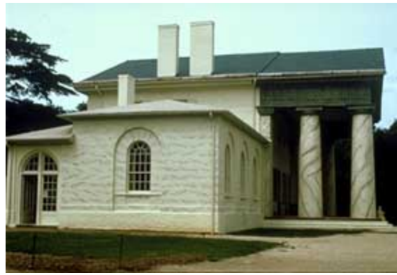
The stucco finish on Arlington House, Arlington, Virginia, was marbled in the 1850s, approximately 30 years after it was built. Photo: NPS files.
