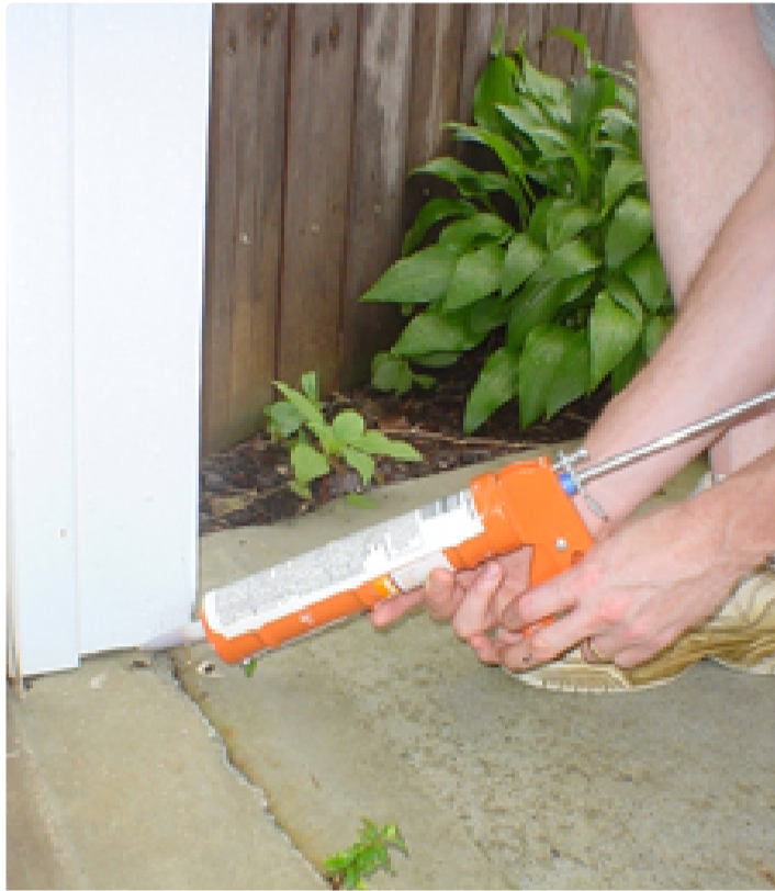
Sealing holes on the exterior of a house.
