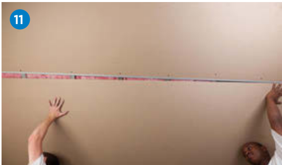
11 Install the next RhinoBoard 6.4mm. Repeat steps 9 and 10 until entire area is covered
