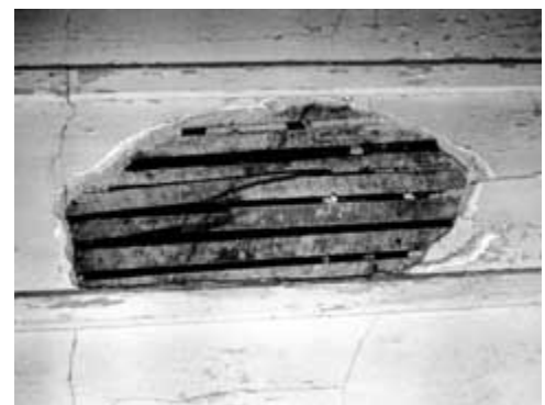
This beaded ceiling in one of the bedrooms of the 1847 Lockwood House, Harpers Ferry, West Virginia, is missing portions of plaster due to broken keys. Photo: NPS files.
