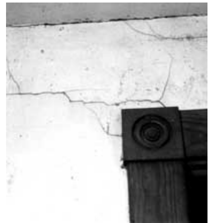
Stress cracks in plaster over a kitchen door frame can be repaired using fiberglass mesh tape and joint compound.
