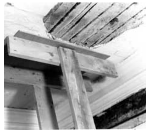
When ceiling repairs are made with wet plaster or with an injected adhesive mixture, the old loose plaster must be supported with a plywood brace until re-keying is complete. Photo: John Leeke.
