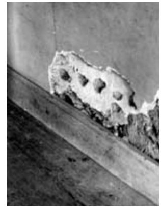
The builders of this mid-18th century house installed the baseboard molding first, then applied a mud and horse hair plaster. Lime was used for the finish plaster. Photo: NPS files.
