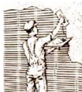
Plasterers applying rough and finish coats of plaster. Drawing: From the "Book of Trades.
