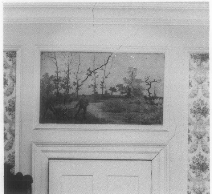
Fig. 12. Settlement caused stress cracking through both flat wall and ornamental plaster. Repairs to the cornice molding involve chamfering the stress cracks to a "V groove" and patching with a mixture of gypsum and lime. The cornice can be countersunk-screwed to its substrate to prevent further movement. Screw heads are then plastered over. The crack running through the painting will need to be filled carefully, and the painting restored by a trained conservator. Photo: Jack E. Boucher, Historic American Buildings Survey.
