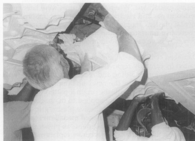
Fig. 23. A pre-cast coffer is lifted into place to abut adjacent panels. Tie wire will be fastened to the channel irons and the superstructure above, twisted to level, and finally wadded with wood fiber soaked in plaster to prevent the wire from stretching. Photo: David Flaharty.
