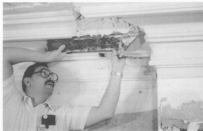
Fig. 5. Miterring a Plain-Run Cornice. Miterring requires great dexterity using the miter rod. In this case, a return at a chimney breast is tooled using an infill of gypsum and lime. Internal and external miters are required with the internal being the most difficult. Another method is to run a length of cornice (using the same blade) on a bench and set it in place, later to point the joints. Photo: Old-House Journal.
