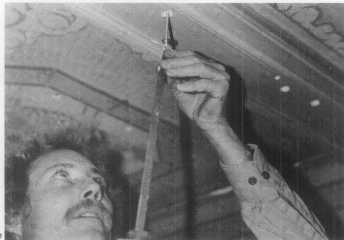
Fig. 17 (a) Where this ceiling was suffering from structural failure, the first step was to shore it up from below. (b) Toggle bolts were used to reattach the plaster molding to the ceiling joists. The ceiling was then patched with gypsum and lime, prior to restoring the significant paint finishes. Photos: National Park Service files.
