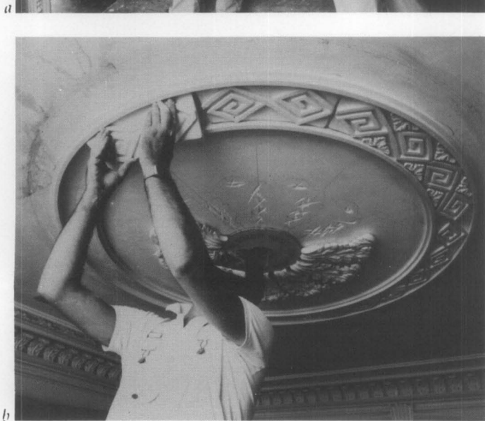
Fig. 7. Running and Enriching a Ceiling Medallion. The method of running and enriching a ceiling medallion remains the same today. (a) First, a plain-run surround is spun from a pivot point centered in the ceiling field. (b) Ornament layout is determined using plane geometric principles; segmented locations are deeply scratched to provide a rough surface for adequate bonding using plaster as an adhesive. Historically, cast enrichments could be bought from local suppliers and set individually, allowing architects to compose medallions to suit room dimensions and period motifs. Photos: Peter Sanders.
