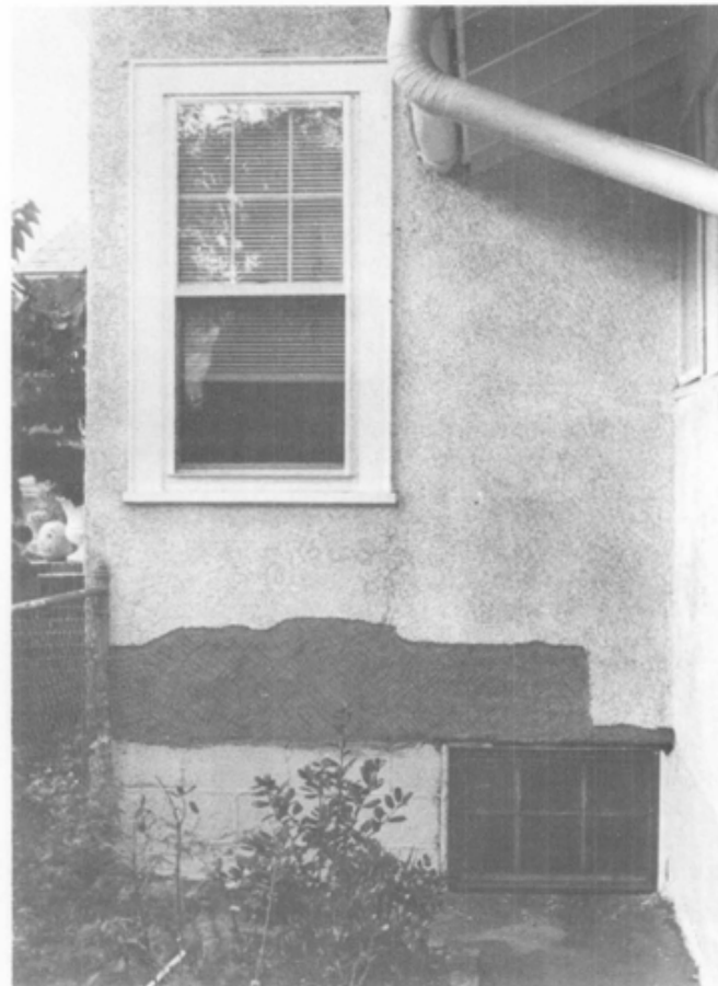
Fig. 15. (a) After reattaching any loose wood lath to the furring strips underneath, the area to be patched has been cleaned, the lath thoroughly wetted, and (b) the first coat of stucco has been applied and scratched to provide a key to hold the second layer of stucco. Photos: Betsy Chittenden.
