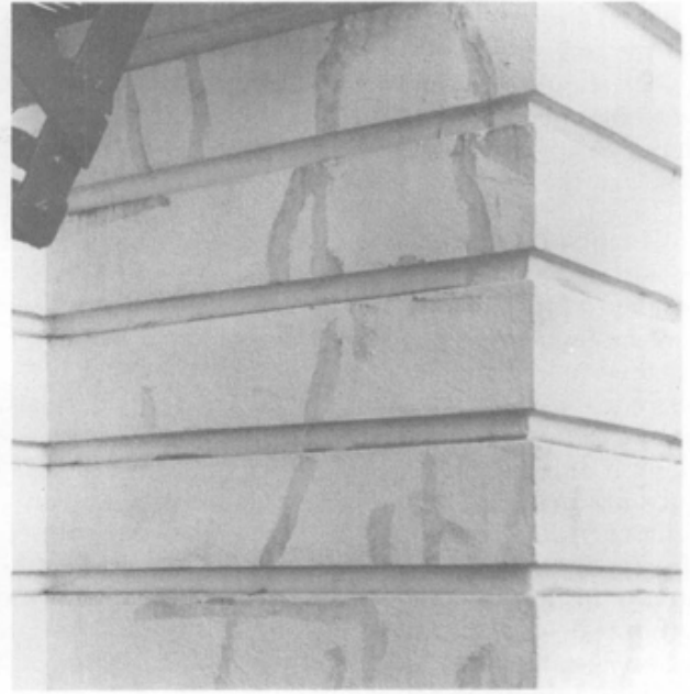
Fig. 13. (a) In preparation for repainting, hairline cracks on this Mediterranean style stucco apartment building were filled with a commercial caulking compound; (b) dirt is attracted and adheres to the texture of the caulked areas, and a year after painting, these inappropriate repairs are highly obvious. Photos: Anne Grimmer.
