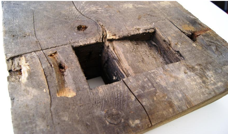
Figure 4 – The mortice
