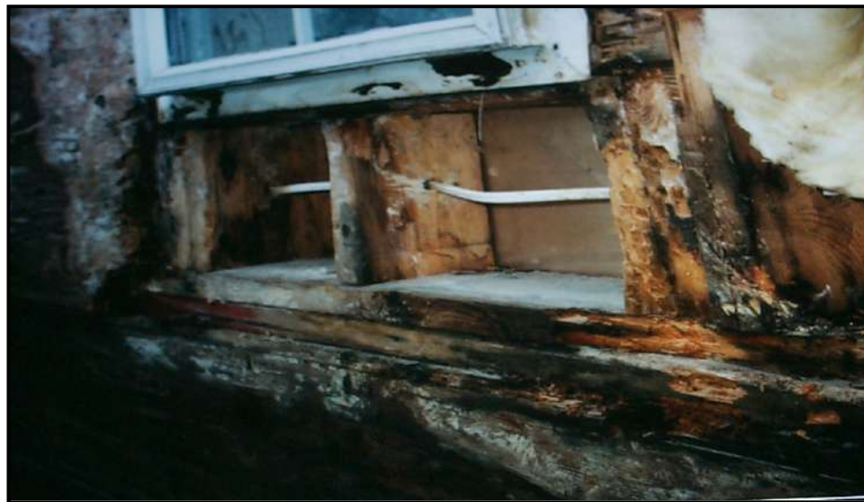
Figure 1 Damage due to moisture inside a wall.
