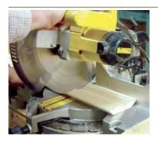
(F) Cut crown moulding (#3 in FIGURE 1) to fit the distance measured between #1 and #2, using simple, straight cuts.
