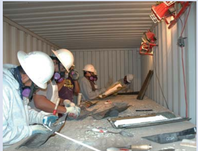
Figure b. On pieces where paint remained after the freezing/flex process, workers carefully hand scraped with chisels to finish the clean-up. Because lead paint was present, workers were required to wear NIOSH approved-respirators.
