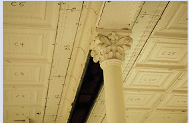
Figure a. Removal began with documenting the pieces within each room, numbering and noting their precise location on a drawing. It was important that the pieces were marked in such a way that the numbers would remain legible throughout the cleaning and reinstallation process.
