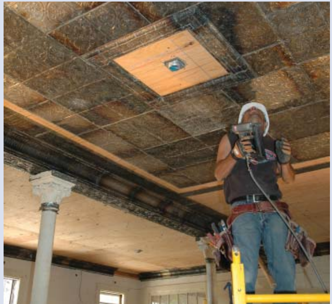
Figure d. Following the installation of the sound-proofing materials and drywall, the pressed-metal pieces were reinstalled using brads and a pneumatic gun. Matching the numbered pieces to the placement diagrams made the reinstallation easy.
