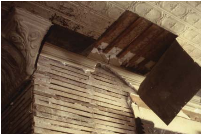
Prior to repair, a section of the pressed metal was removed to expose the condition of the plaster and lath and to document the earlier finish. (Photo: Kaaren Staveteig, NPS)
