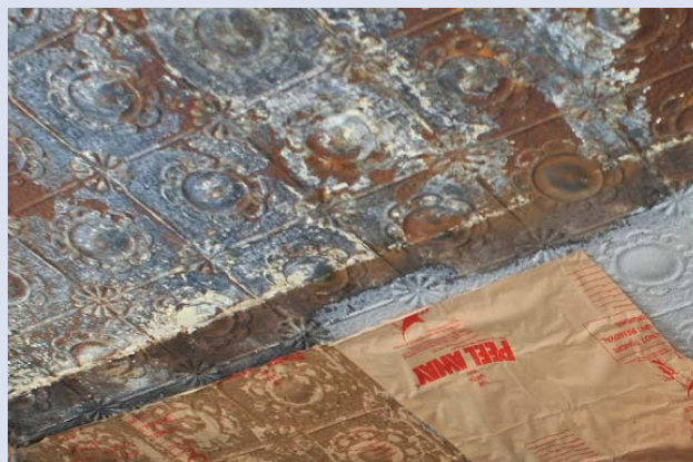
After applying a solvent-based paint to the metal, a laminated cloth/paper is applied during the chemical-peel process. (Photo: NPS)
