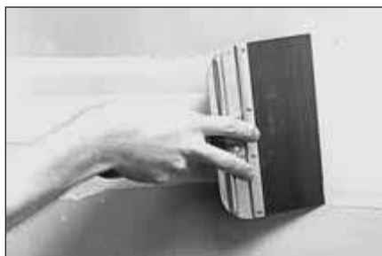
2. First Finishing Coat
