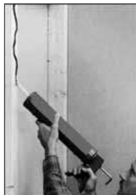
ADHESIVE/NAIL-ON Ideal for prefinished boards.
