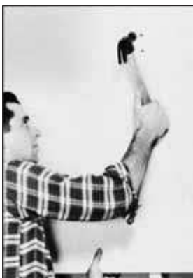
DOUBLE NAILING Minimizes nail-pop.
