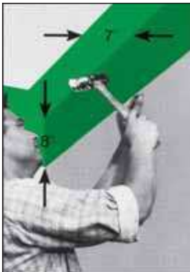
FLOATING ANGLES No nails in shaded area.
