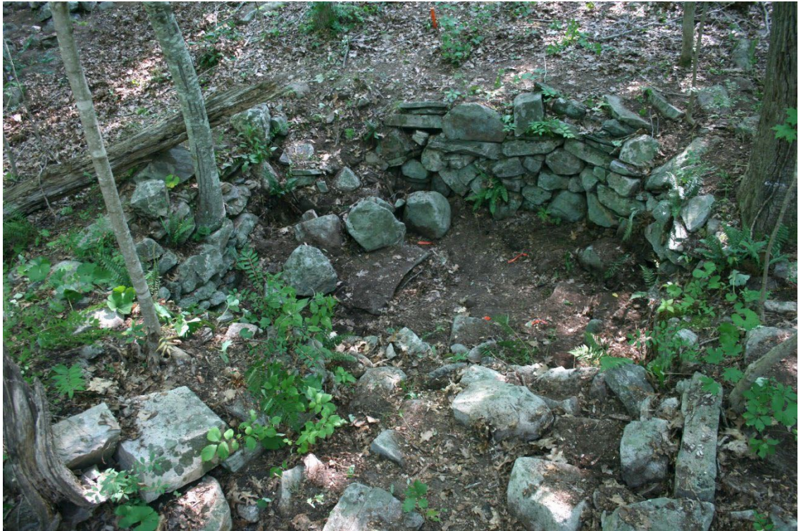
Figure 20. Site 102-82 Stone-Lined Cellar, View from Southwest Corner of Foundation, Looking Northeast. Courtesy of Stephen Silliman
