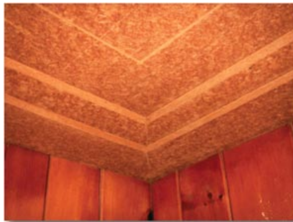
Figure 3—This fiberboard ceiling in the Butte Falls Ranger Station (Rogue River-Siskiyou National Forest, Pacific Northwest Region) has been carved into a decorative pattern. The ceiling is the natural brown color of the wood pulp from which it was manufactured.
