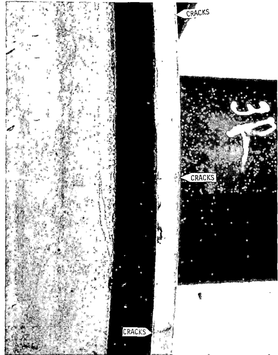
Fig. 4, Typical Wheel Flange Cracks
