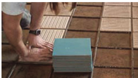
Figure 3.5.1 – Negative Cast Method – Tiles are pressed finish face down into molds. Notice the key backed (dove tails) configuration of the tile.
