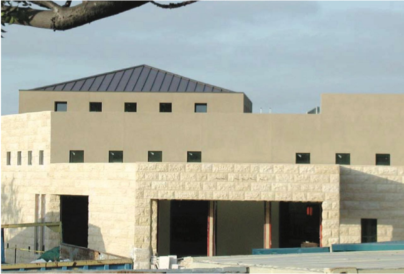
Photo: Project — Temple Emanuel, San Diego, CA 2008, Contractor: Howard's Rug Company, San Diego, CA Description: Jerusalem Gold limestone facade installed with 254 Platinum over 9235 Waterproofing Membrane.
