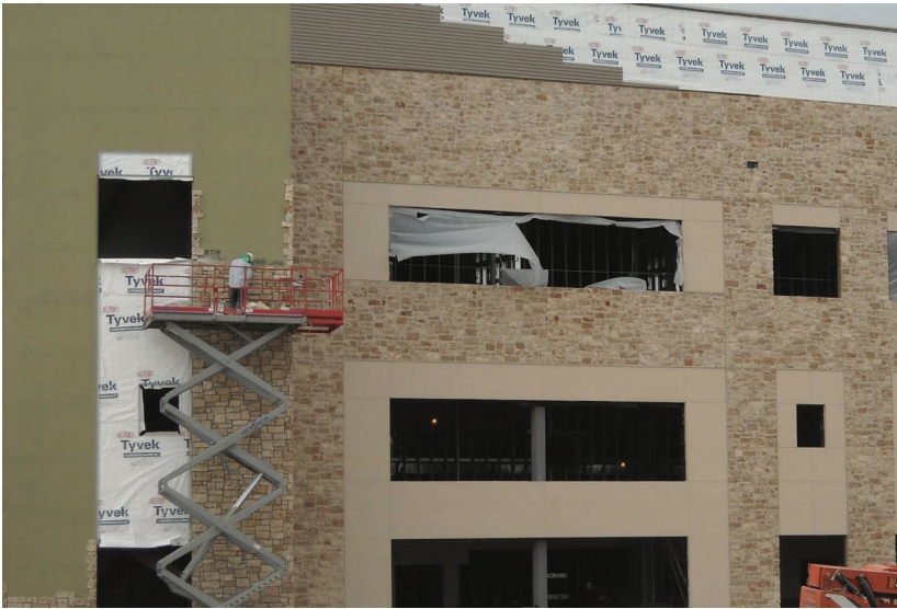
Photo: Project — Cedar Park Center, Cedar Park, TX 2010, Contractor: Trinity Drywall & Plastering Systems, Ft. Worth, TX. Description: Manufactured Veneer Masonry installed with Masonry Veneer Installation System (MVIS™).
