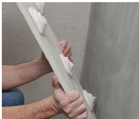
Figure 7.3.2 – Spot bonding with LATAPOXY 310 Stone Adhesive.
