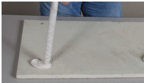
Figure 7.4.6 — Dabs of LATAPOXY® 310 Rapid Stone Adhesive in cartridge packs being applied using the LATAPOXY 310 Cordless Mixer.
