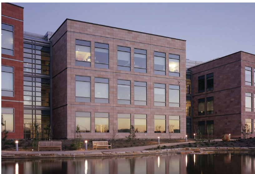
Photo: Project-Biogen Idec, San Diego, CA 2005, Architect: HOK, Culver City, CA; Stone Contractor: Kloser Tile, Chula Vista, CA. Description: Indian sandstone veneer over cement render over steel framing and exterior rated sheathing.
