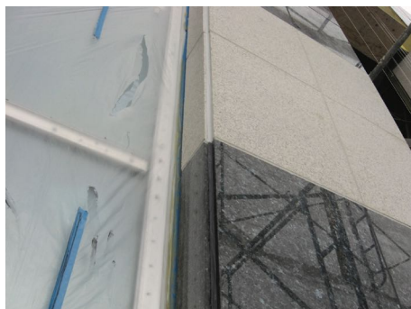
Figure 4.2.7 — Use of movement joints as an integral facade design element®.
