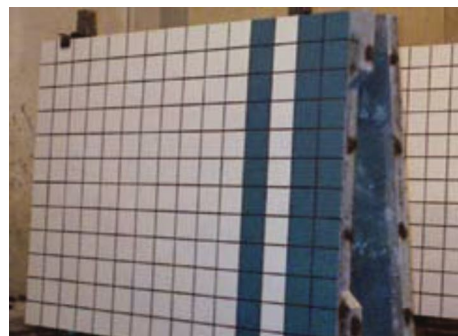
Figures 3.5.4 – The grouted panels are then stored and allowed to cure before being transported to the job site for installation of the panels.
