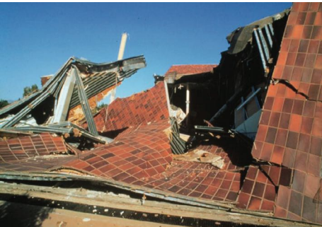
Figure 7.1.2 — High adhesive shear and tensile strength to resist seismic movement. 15 Tile remains adhered even after severe shear stress from seismic activity caused structural failure.
