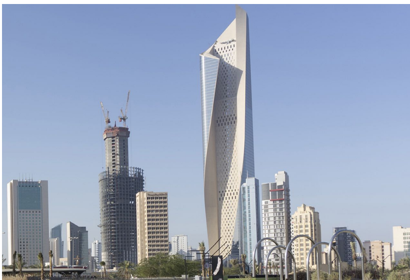
Photo: Project-Al Hamra Building, Kuwait City, Kuwait 2009, Architect: Skidmore, Owings Merrill, Chicago, IL; World's Tallest Direct Adhered Façade Installation. Description: 220,000 ft 2 (20,370 m 2 ) of trencadis limestone veneer installed with 254 Platinum over poured concrete on the 1,350' (414 m) high tower with a 130° turn in the structure.
