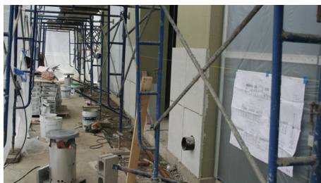
Figure 5.3.3a and 5.3.3b — Proper protection of an exterior façade tile or stone installation during winter months in cold climate.
