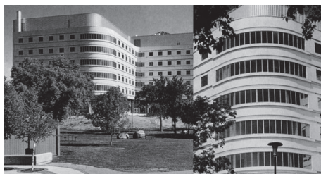
Figure 3.7.2 – Saskatoon City Hospital – Ceramic tile clad pre-cast concrete panels.
