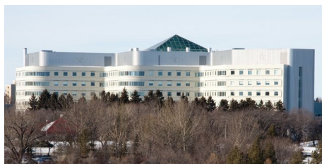
Figure 3.7.1 – Saskatoon City Hospital – Ceramic tile clad pre-cast concrete panels.
