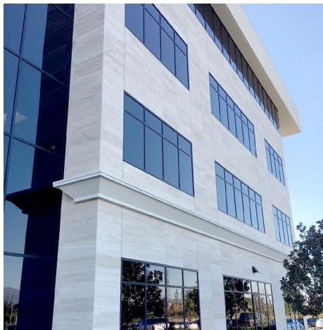
Figure 1.3.2 Large-format travertine natural stone facade—City of Industry, CA, USA.
