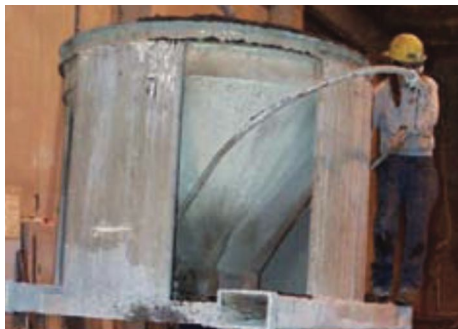
Figure 3.5.2 – Negative Cast Method – Concrete is poured and vibrated over the panels. A slurry bond coat of 211 Powder mixed with 3701 Mortar Admix can be used as a bonding agent between the tile backs and the concrete pour in this method.
