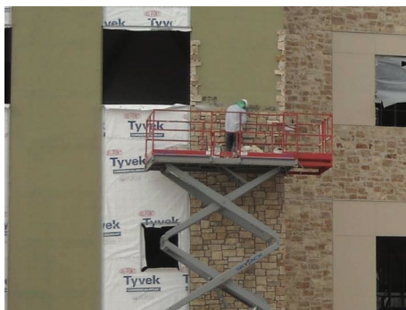
Figure 6.4.1 — AMSMV Installation Over MVIS™ Air & Water Barrier
