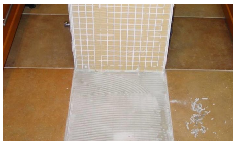
Figure 7.4.9 — Example of incomplete bedding caused by omission of back buttering.
