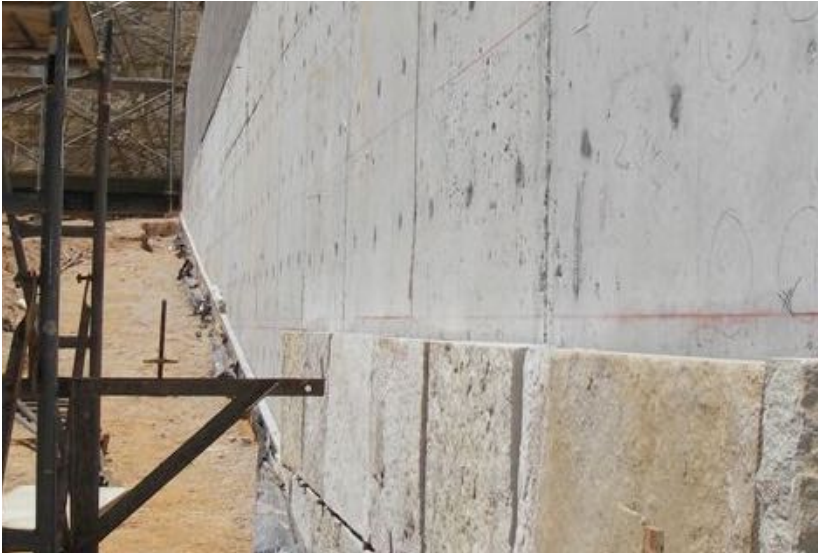
Photo: Project-Umstead Hotel, Research Triangle Park, NC 2006, Architect: Three Architecture, Inc, Dallas, TX; Stone Contractor: David Allen Co., Raleigh, NC. Description: 20" x 30" (510 mm x 762 mm) limestone installed with LATAPOXY® 310 Stone Adhesive.
